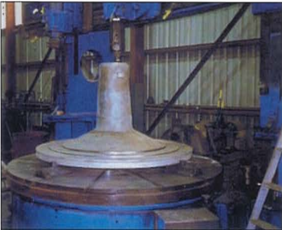
REPAIRING BUSHING FIT & REPLACING WEAR PLATES IN 73" MILL BOTTOM
