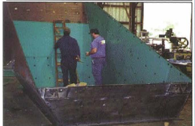
SCREEN CHUTES BEING LINED WITH UHMW
